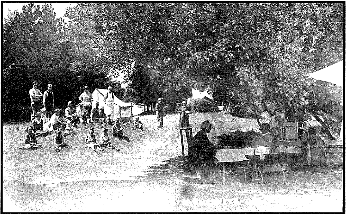
Patton postcard view of the Campgrounds at Manzanita. Camping meant renting a tent with a wooden floor and a woodstove. Campers used communal outhouses and drew water from on-site wells.
