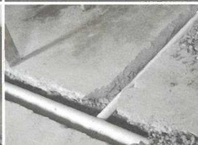
DRAIN PIPES INSTALLED
