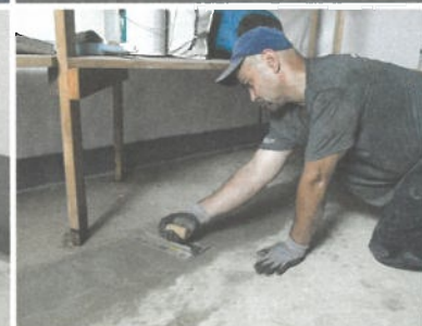
FLOOR RE-CONCRETED
