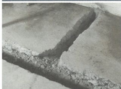
DRAIN TRENCH INSTALLED
