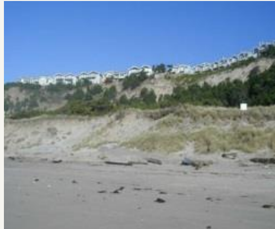
Figure 31. Erosion at “The Capes” Condominiums, Oceanside, Oregon
