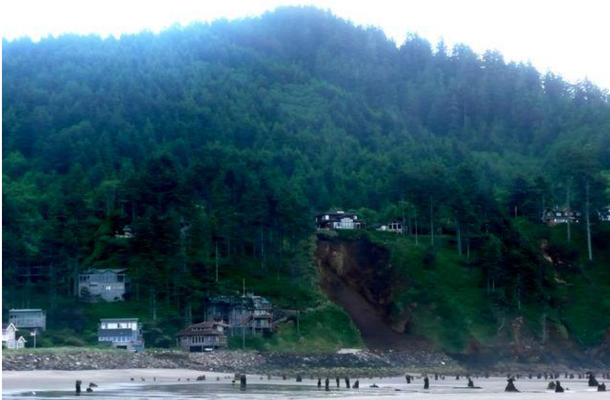
Figure 63. Landslide in Tillamook County
