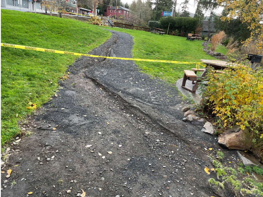
Waterfront Park- Path has divots, holes, and tripping hazards.
