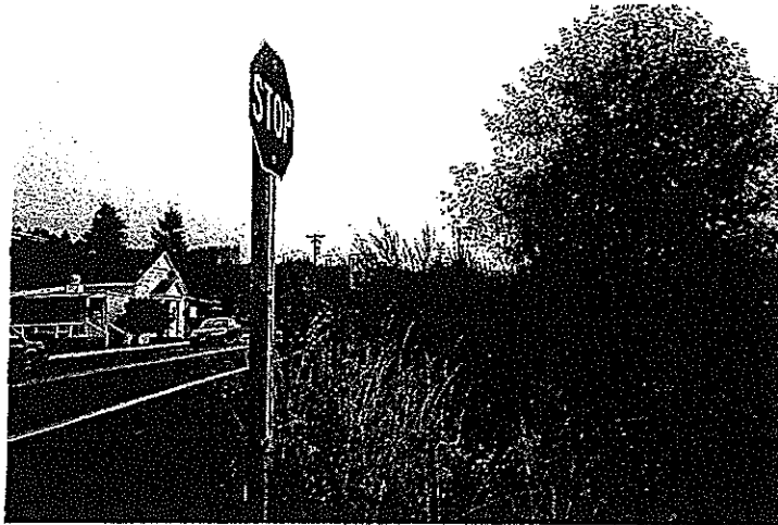
Sight distance (SD) looking south along Hwy 101 from Hemlock Street (SD blocked due to vegetation)
